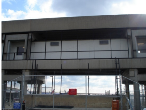
Figure 1: Temporary Connector Bridge Construction
